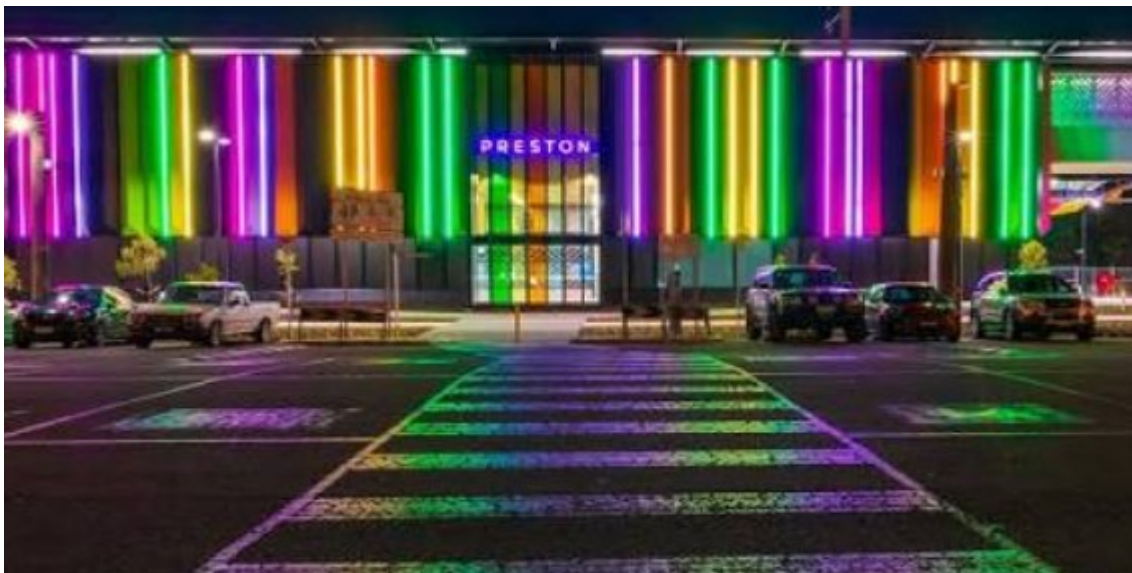
Image 27 Preston Station East Side as seen from Preston Market Car Park at night.
