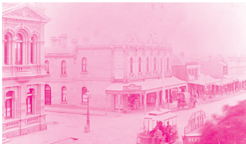
Cable Tram, High Street Northcote
